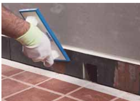
12. Bond on the skirting boards and grout the vertical joints
