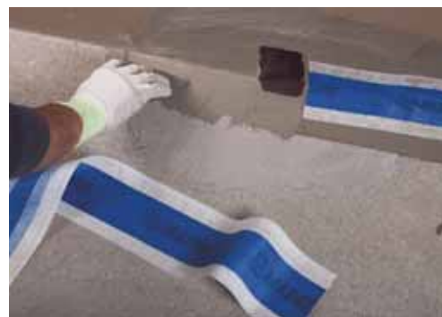
7. Apply the first coat of MAPEI waterproofing product on the clean, dry fillet between the horizontal and vertical surfaces
