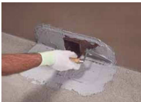
4. Spread on a second coat of Adesilex PG4 fresh on fresh to completely cover Drain Front
