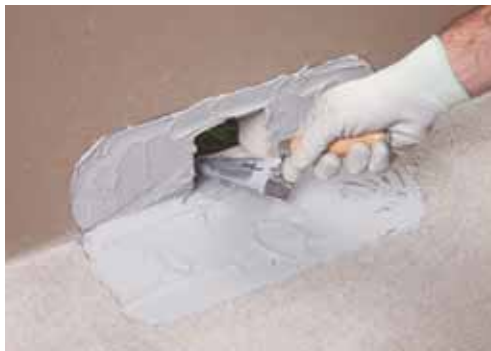
2. Spread on an even layer of Adesilex PG4 two-component, thixotropic epoxy adhesive with a smooth spatula on the clean, dry substrate
