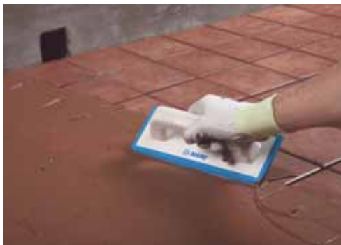
11. After applying the MAPEI waterproofing product according to the relative Technical Data Sheet, bond on the floor coating and grout the joints
