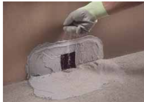
5. Smooth over with a flat trowel and, while the product is still fresh, sprinkle on a layer of 0.5 spheroid quartz to form a rough layer to help the specified MAPEI waterproofing product form a good bond
