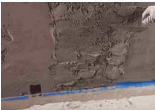
10. Apply a new layer of render on the parapet, or repair the old render removed before carrying out installation in the case of old structures
