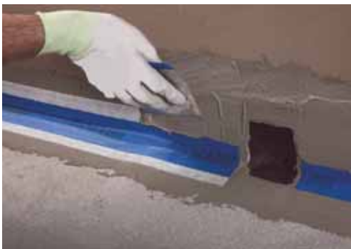
8. Lay on Mapeband by pressing along the sides, making sure there are no creases or air bubbles
