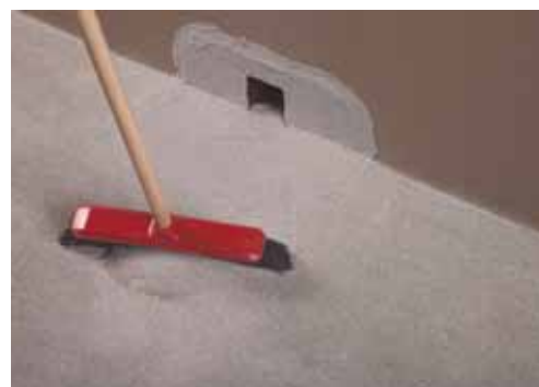
6. Once the reticulation process of AdesilexPG4 has been completed, remove any loose quartz
