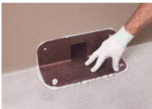
3. Place Drain Front in position and press down lightly so that it is embedded in Adesilex PG4
