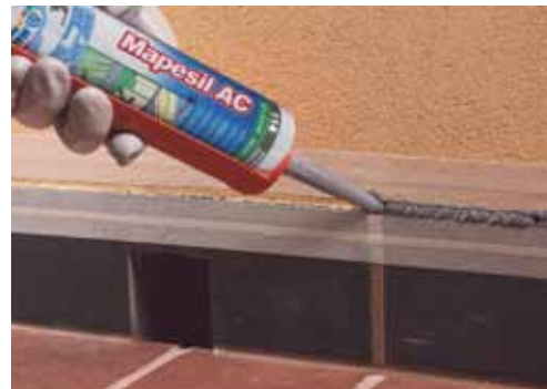
13. Seal with Mapefil AC in correspondence with the skirting board-wall fillet joint
