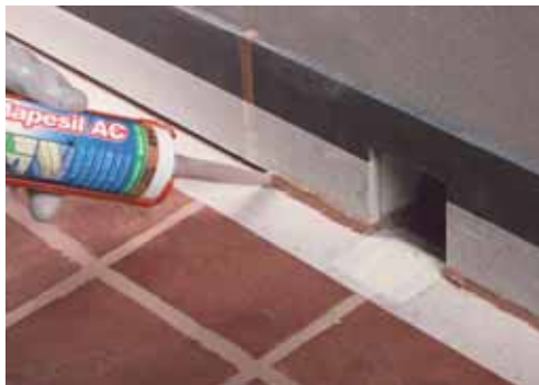
13. Seal with Mapefil AC in correspondence with the skirting board-wall fillet joint
