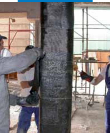
Impregnation with "wet system" of MapeWrap C UNI-AX HM with MapeWrap 31
